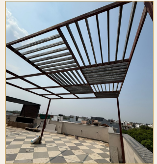
MS I-beam and purlin structure erected
